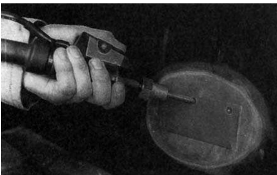
Figure 10.22 Single-sided spot welding used in panel repair ( Stanners Ltd )
