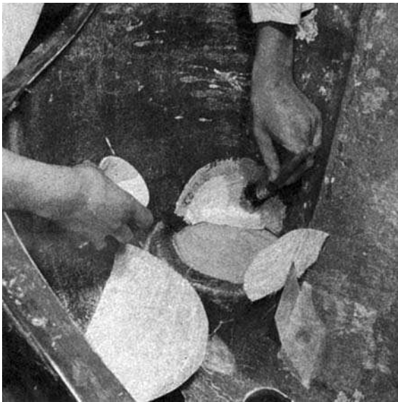
Figure 16.39 Applying chopped strand mat
