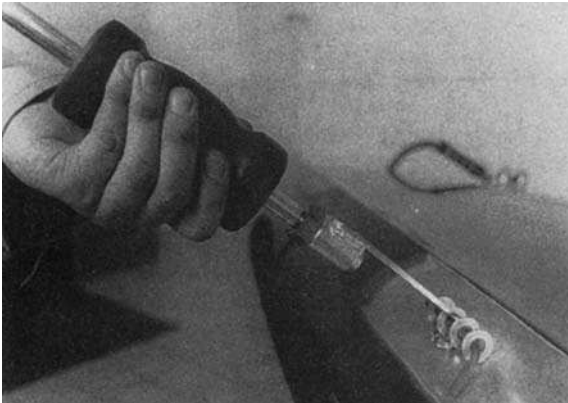
Figure 13.66 Pulling damage out using hook and slide hammer ( Stanners Ltd )
