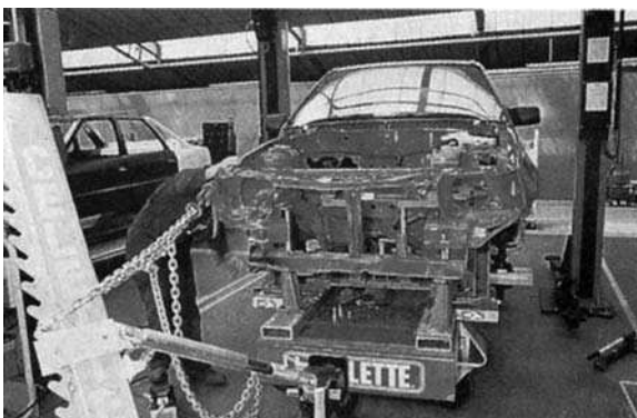
Figure 14.82 Vehicle on jig being pulled before cutting out damaged sections ( Motor Insurance Repair Research Centre )
