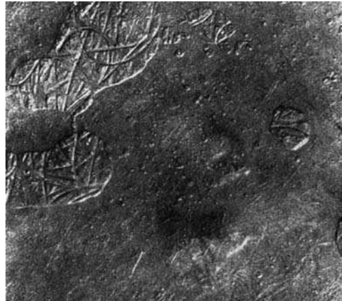
Figure 16.50 Severe blisters ( Scott Bader Co. Ltd )
