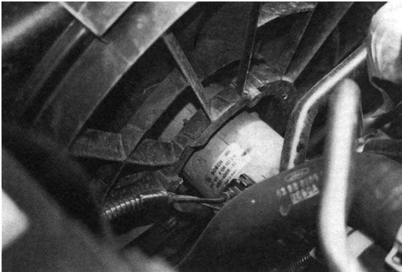
Figure 9.23 Cooling fan motor
